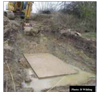
Fig 2: Concrete pad for base
