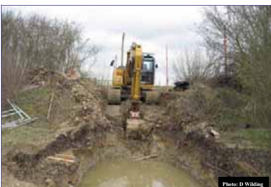
Fig 3: Installation of tilting weir
