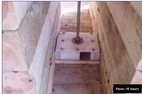
Fig 2: The impellor unit
