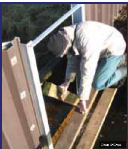
Photo: N Droy Fig 3: Inserting a dropboard
