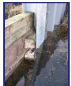
Fig 2: Dropboards and wooden chocks
