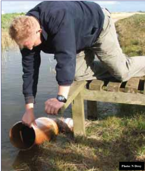
Fig 8: Adjustment of water levels using 'Osma pipe' right angled bend
