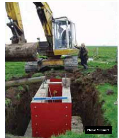
Fig 3: Installing the pump chamber
