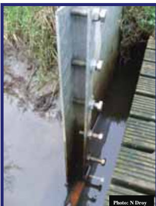
Fig 3: Retaining bolts
