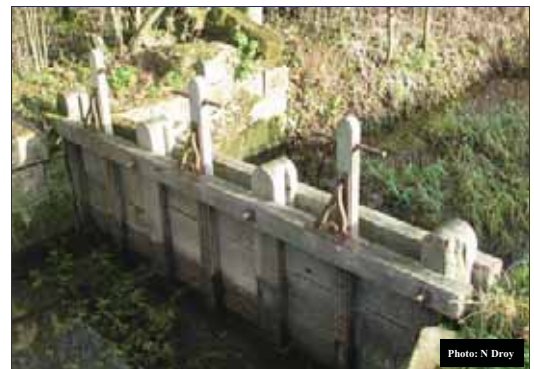
Fig 5: A traditional wooden penstock weir
