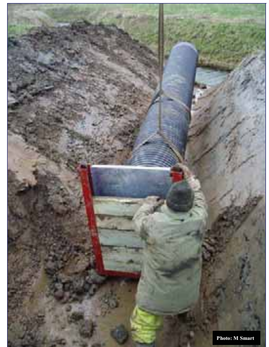
Fig 3: Lowering the sluice unit in to position
