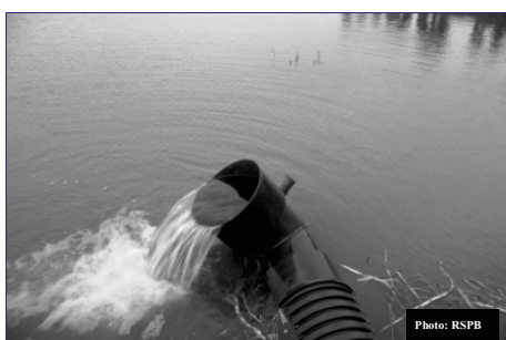
Fig 4: Water flowing through control pipe
