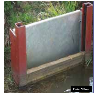
Fig 1: Drop board sluice
