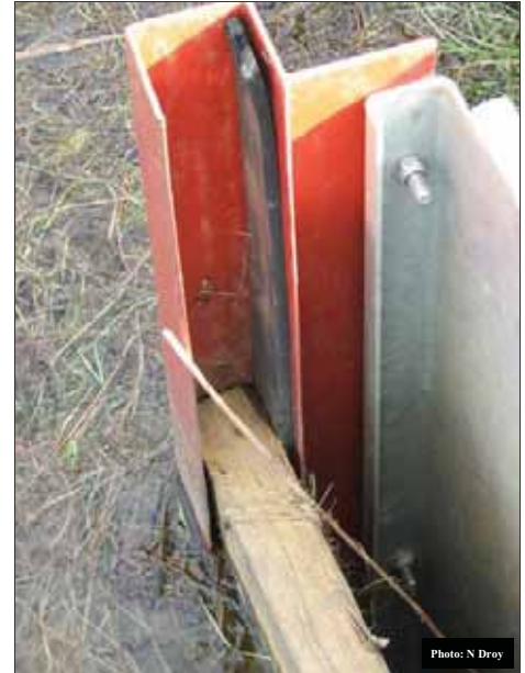
Fig 5: Detail of rubber seal on structure
