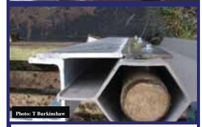
Fig 6: Sluice frame & wooden supports
