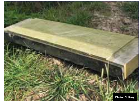
Fig 6: Drop board with rubber seal
