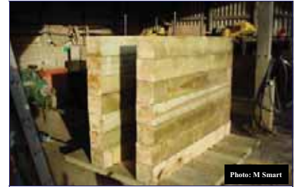
Fig 1: Pump chamber construction
