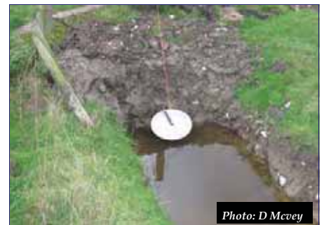
Fig 9: Non return flap valve
