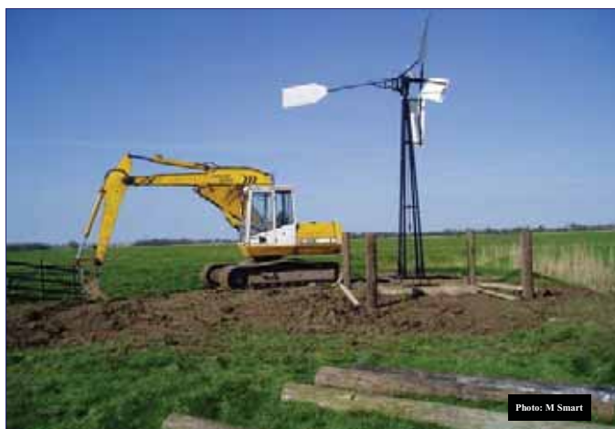
Fig 4: Installation was completed within one day
