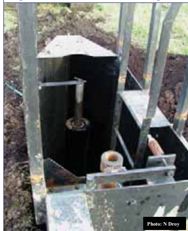
Fig 2: Custom made trenching box
