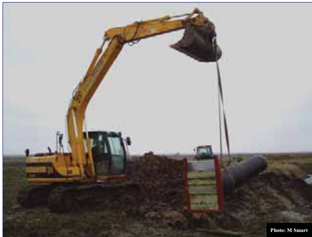
Fig 2: 360 excavator installing sluice structure
