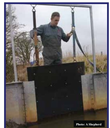
Fig 2: Sluice operation
