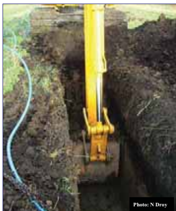
Fig 3: Excavating the trench
