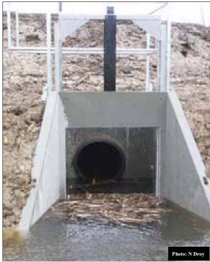
Fig 1: Overflow weir
