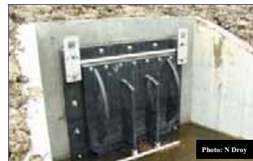
Fig 4: non-return flat valve
