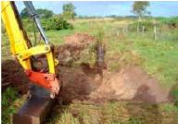
1. Exposing the sub surface tile drain
