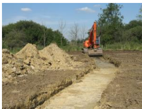
Backfilling the line of the drain with clay, Oxon.
