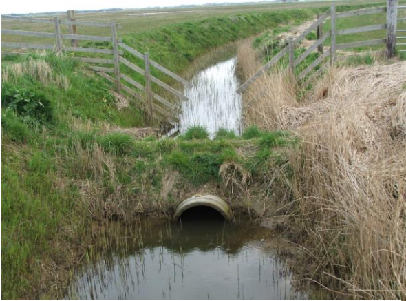
Drainage ditch and bund, Norfolk
