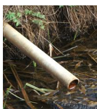
Drainage outfall pipe
