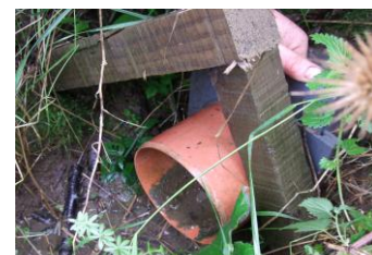
Outfall pipe control, Warwks.
