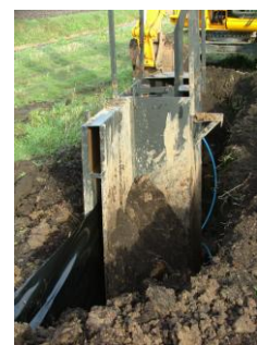
Plastic sheet dispensing from trenching rig, Cambs.
