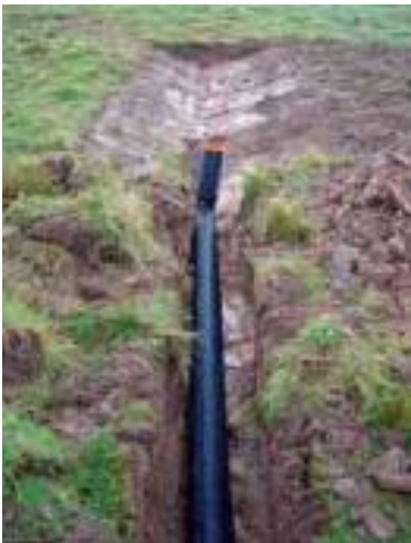
3. New plastic pipe installed with right angles bend control
