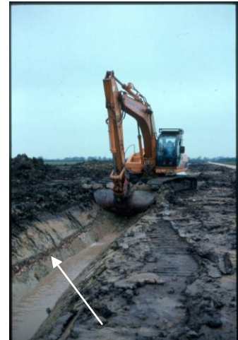
An excavator removing a section of sub surface tile drain, Oxon.
