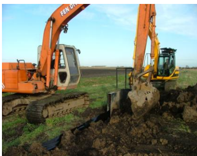
Installing a plastic membrane, Cambs
