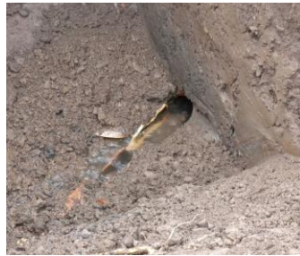
Clay pipe exposed by excavations, Oxon.
