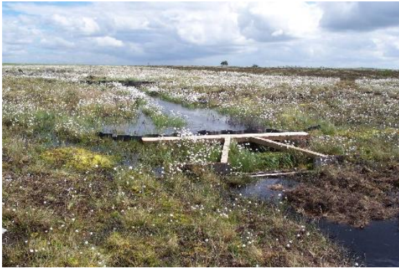
A-frame dam with diagonal timbers linked to the ditch bank – Credit: Andrew McBride, NatureScot
