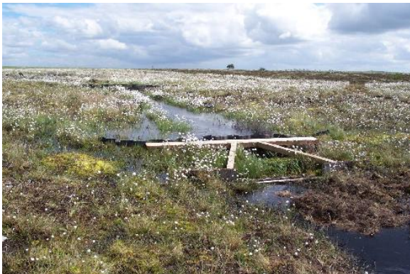
A-frame dam with diagonal timbers linked to the ditch bank – Credit: Andrew McBride, Scottish Natural Heritage
