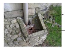
Raised kerbs if properly sealed can prevent contaminated run-off entering a clean water (roof) drain
