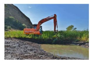
Asymmetrically excavated pond profile providing both depth (right) and gentle gradients (left).
