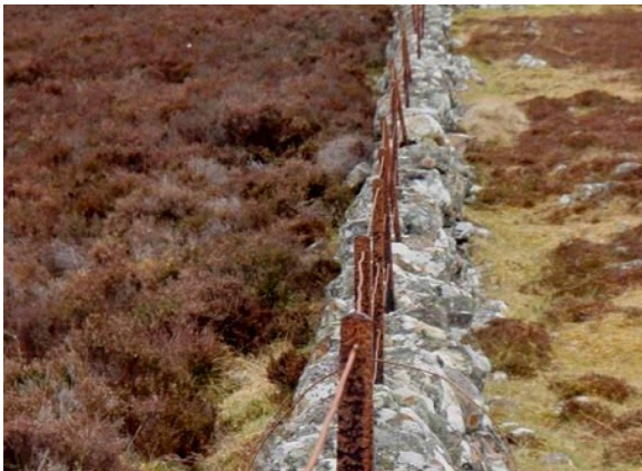
On the right side of the dyke the heather has been suppressed by grazing, and has been replaced by grassy patches – Credit: Graham Sullivan – © NatureScot
